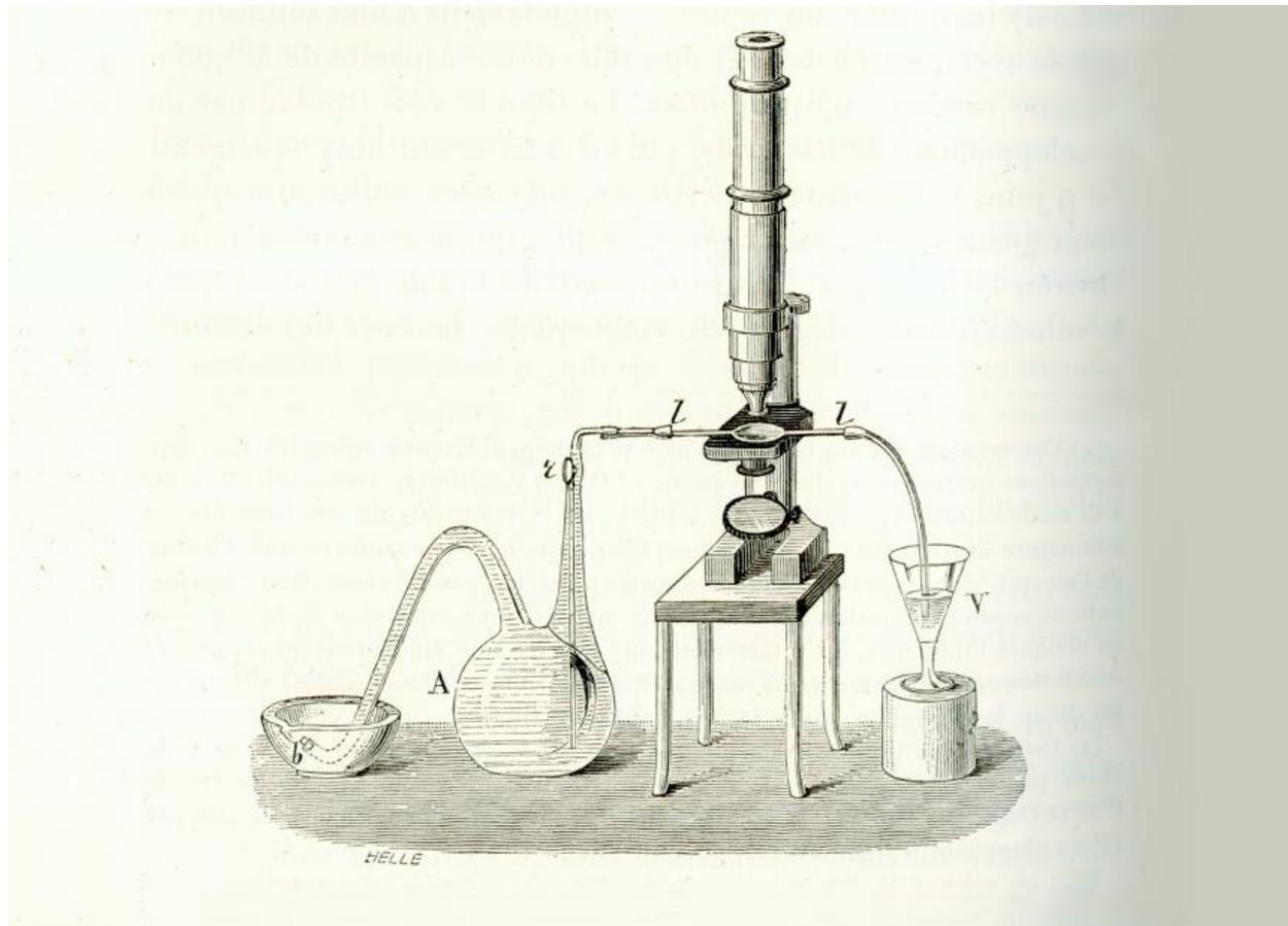
Fig. Equipment used by Pasteur for examination of contamination in Beer fermentation
